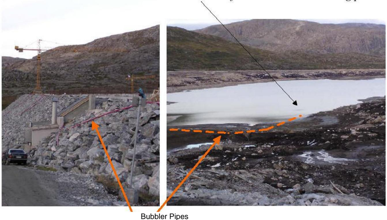
MK4 can measure up to five different pressures sequentially, e.g. water level in the reservoir, pressure drop over a trash rack (to monitor and plan when it has to be cleaned) as well as minimum water flow downstream and leakage water of a filler dam. Up to 500 meter long bubbler tubes can be hooked up to the system. The air supply in most installations comes from a 50 liter 200 bar air bottle which lasts 2 to 5 years depending on the system layout.
